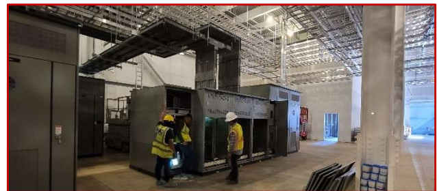
Electrical P anel, B usduct
