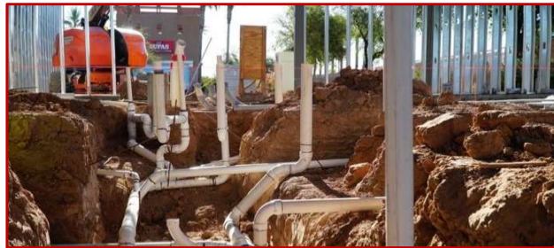
Restroom P lumbing
