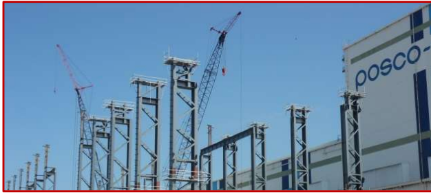
Steel S tructure
