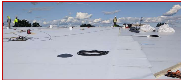
Roofing T PO
